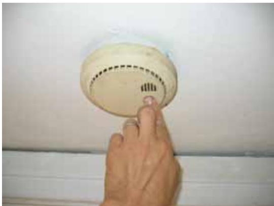
**Smoke Detectors.** After moving in, consider replacing all of the smoke/fire detectors in the entire house. The building should have functioning smoke detectors. Detectors should be wired to a power source and also should contain a battery. Smoke detectors do not last forever. Replace detectors according to manufacturer's recommendations. Test the detectors regularly.
